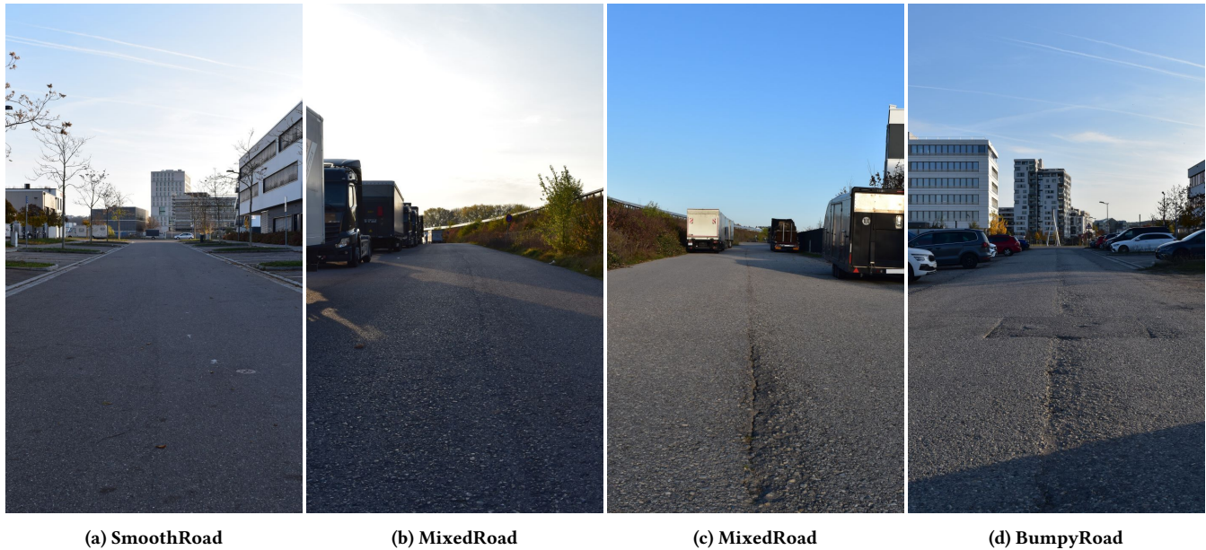
Figure 5: Overview of road types investigated in our study, depicting variations in surface quality.
